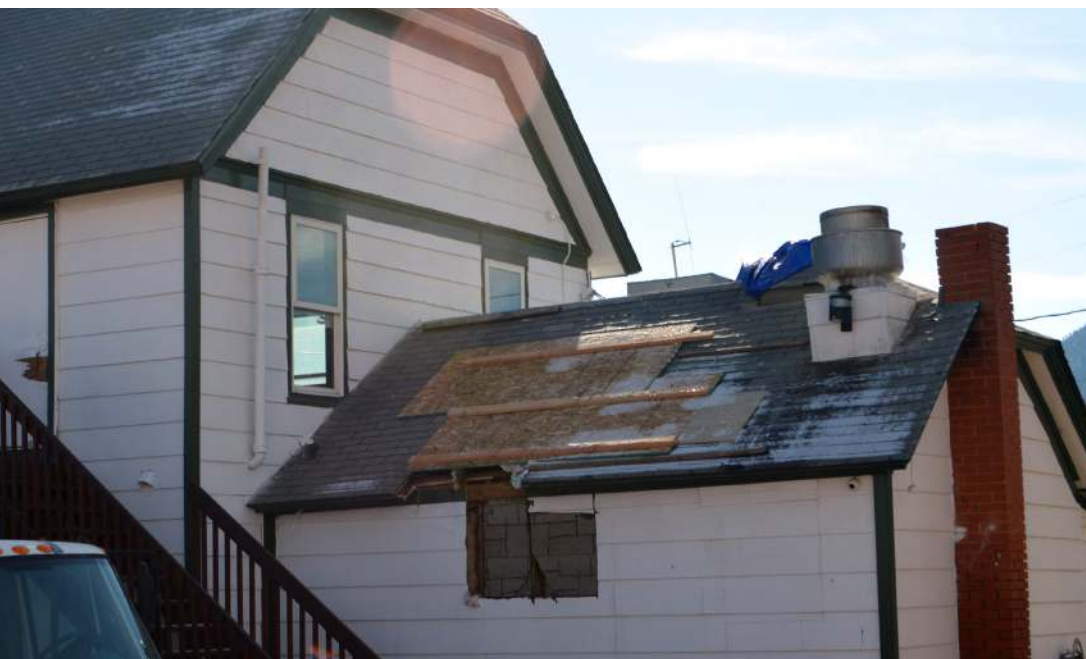
Left: While fighting the fire, the Palmer Lake Volunteer Fire Department had to break part of the kitchen building to allow for flames to escape and to verify that the fire did not exist in the wall. After the fire was extinguished, the staff of O'Malley's boarded up the
